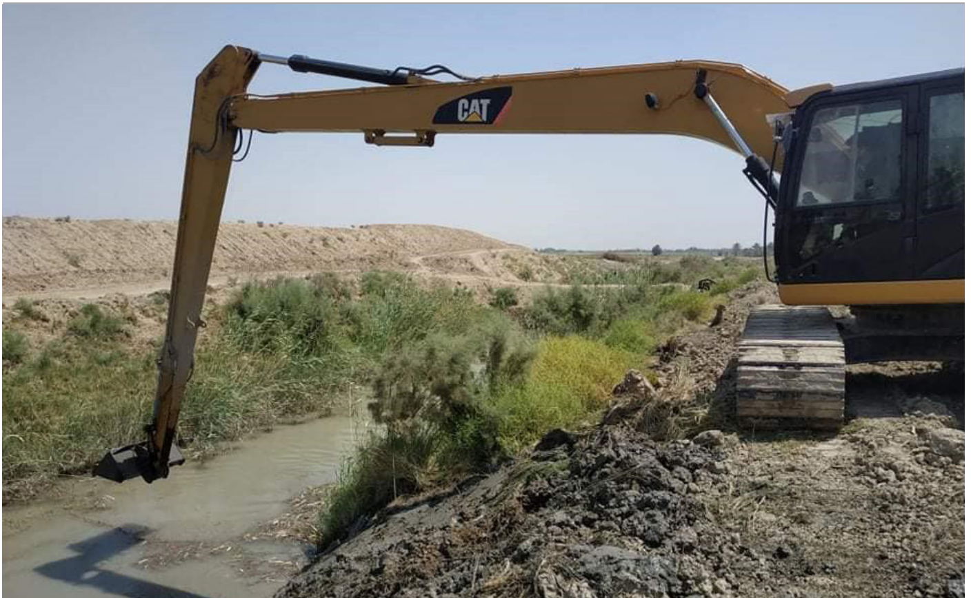
Clearing irrigation channels in Babil Province © Ministry of Water Resources
